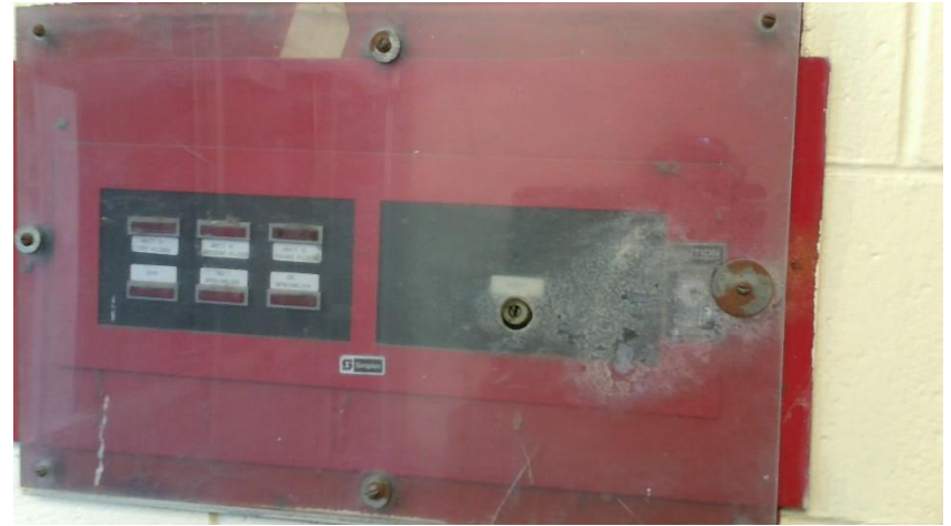
Original Simplex fire alarm system annunciator. Toll Gate High School
