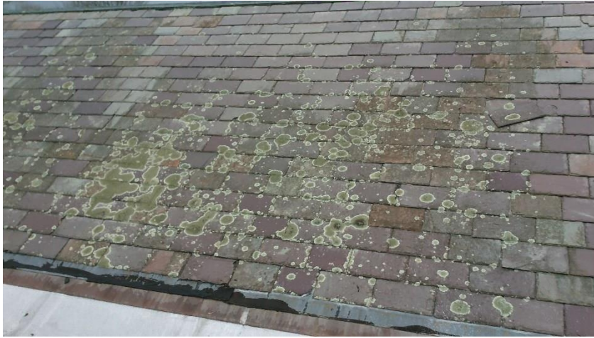
Mold on slate shingle roofing. Peace Dale Elementary School
