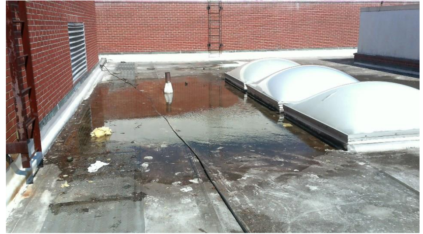
Weathered roofing with significant debris and ponding. Tiverton High School
