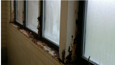
Corroded steel windows East Providence High School
