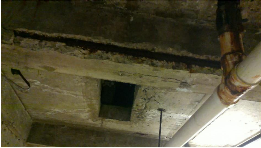
Concrete delamination to the cast in place concrete beams and slabs. East Providence High School
