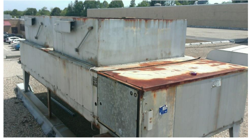
Aged and rusted condensing unit. John F. Deering Middle School
