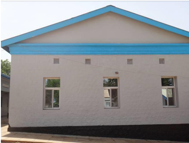
Exterior wall of Surgical block after repainting with weather guard
